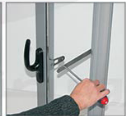
Vent disengaged from limit stop
