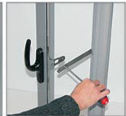
Vent disengaged from limit stop
